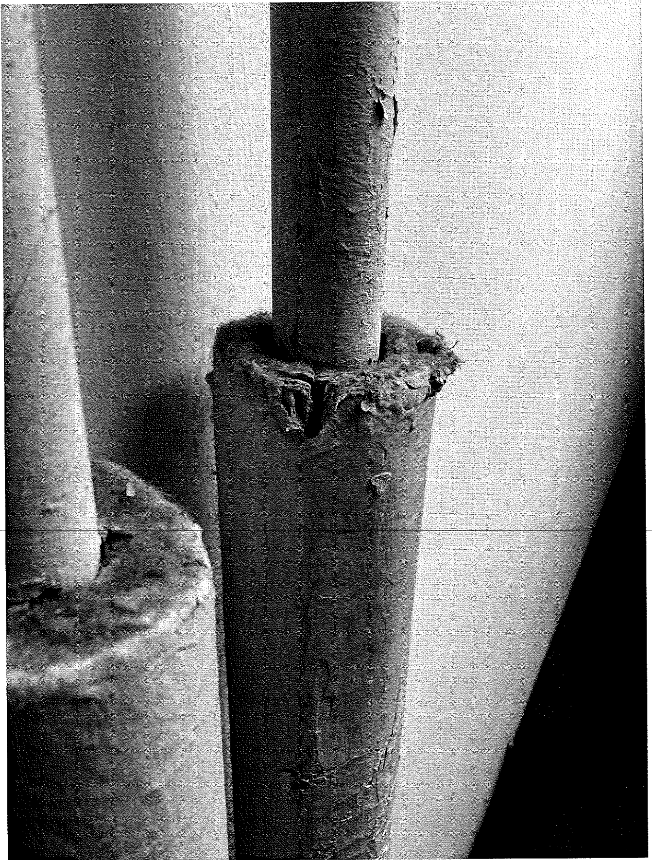
Aircell Pipe Insulation on Heating Lines
